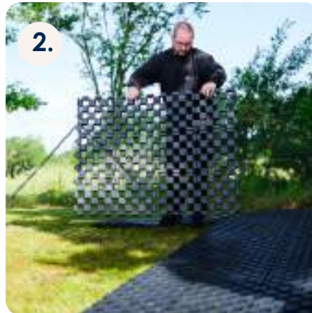
Lay out the Terra-Grid E® 35 panels
