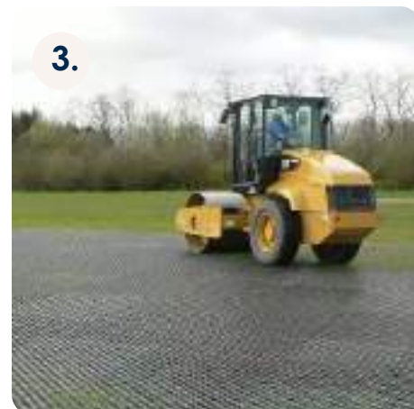
3. Press the panels firmly into the grass
