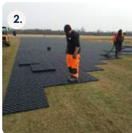
2. Lay out the Terra-Grid E® 35 panels
